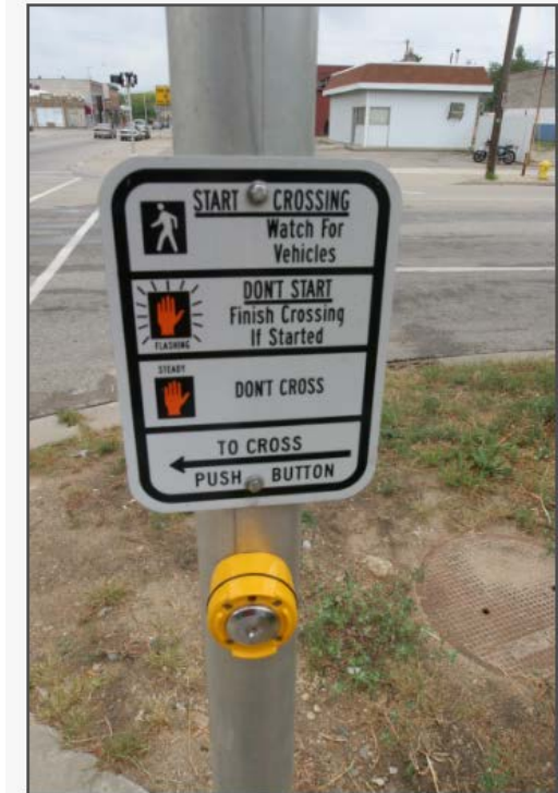
A pedestrian push button provides allows pedestrians to activate a pedestrian signal and reassure pedestrians that they will receive a crossing indication. Source: pedbikeimages.com - Dan Burden (2006)
