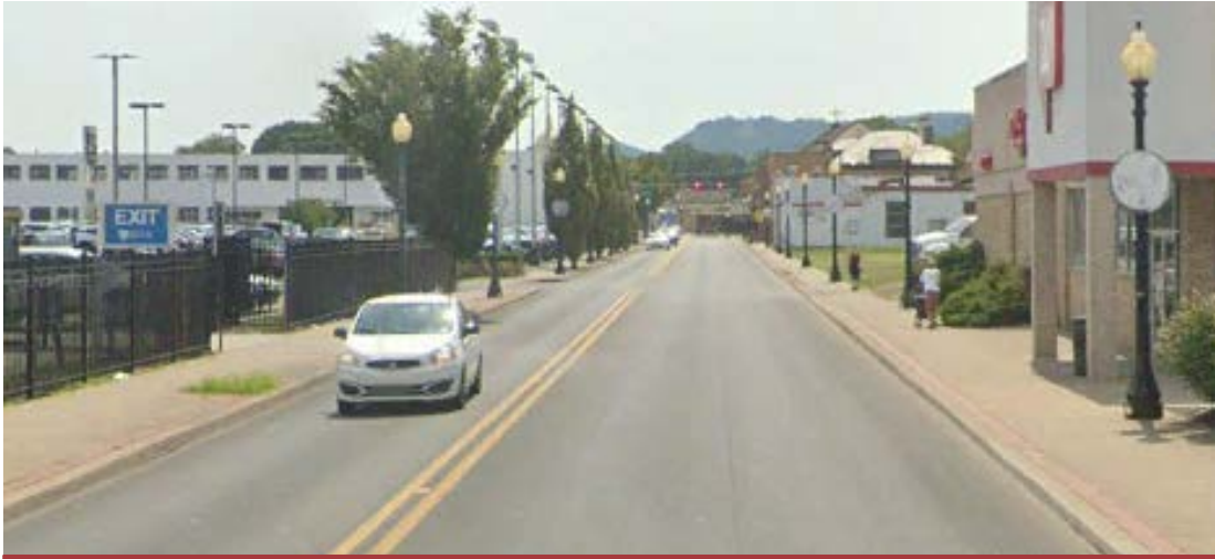
Washington Street between Morris Street and Bradford Street
